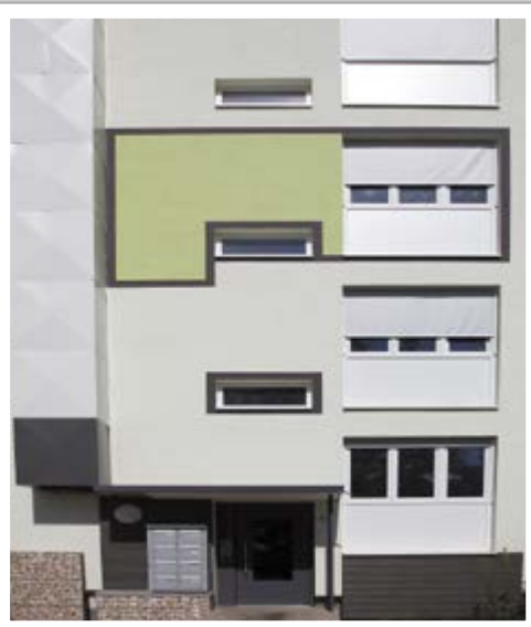
Réhabilitation, Dole, 39, © ADEME Studio Schoolmeesters
