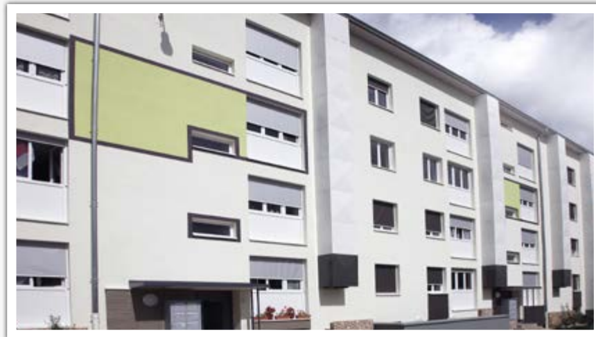
Réhabilitation, Dole, 39, © ADEME Studio Schoolmeesters
